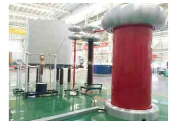
500kV 0.3A for Reactor Testing
